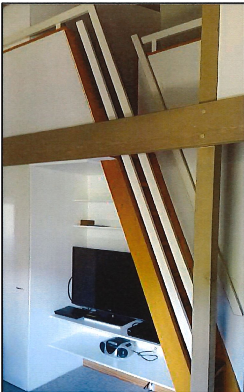
Figure 3: Example of a ladder stair within Riverside Cabins and a completed stair
